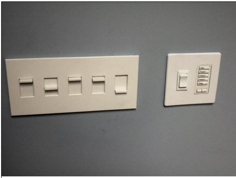
*Figure 3: Typical Room Control Panel Example\* (note that the low-voltage projection screen switch module and window shade control module are segregated from the high-voltage lighting controls)*
